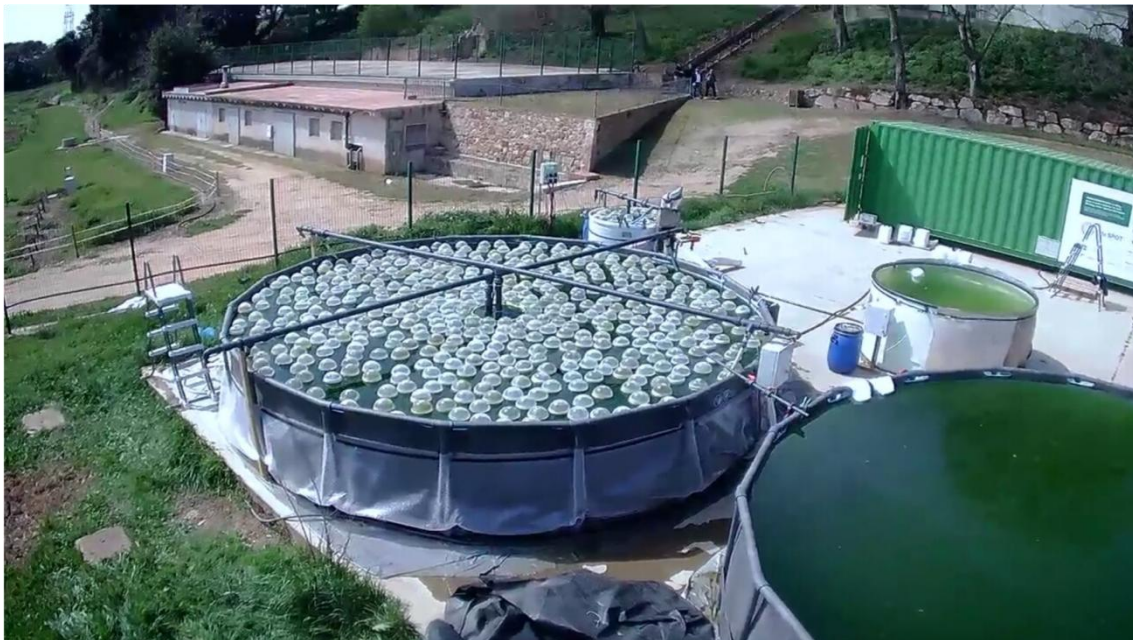
Life SPOT pilot plant at Torre Marimon facilities, Caldes de Montbui
